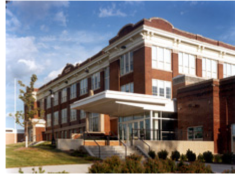
Fig 45 restored elementary school
